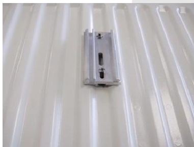
7-11 INSTALLATION OF HEAT CONDUCTOR GUARD
